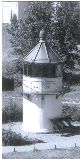
Ranzow Lighthouse once stood several miles southeast of Kap Arkona but was moved to the cape when a modern light replaced it. This design is typical of many small, hut-style lights in Germany. Author photo.
