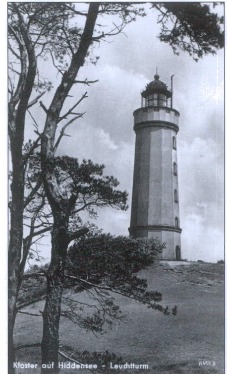
Dornbush Light is the sentinel of the enchanting isle of Hiddensee, on the west side of Rügen Island. The tower was round when first built in 1888. In 1927 it was encased in an octagonal wall to strengthen it. Bird repellents can be seen on the cupola. Collection of Michel Forand.
