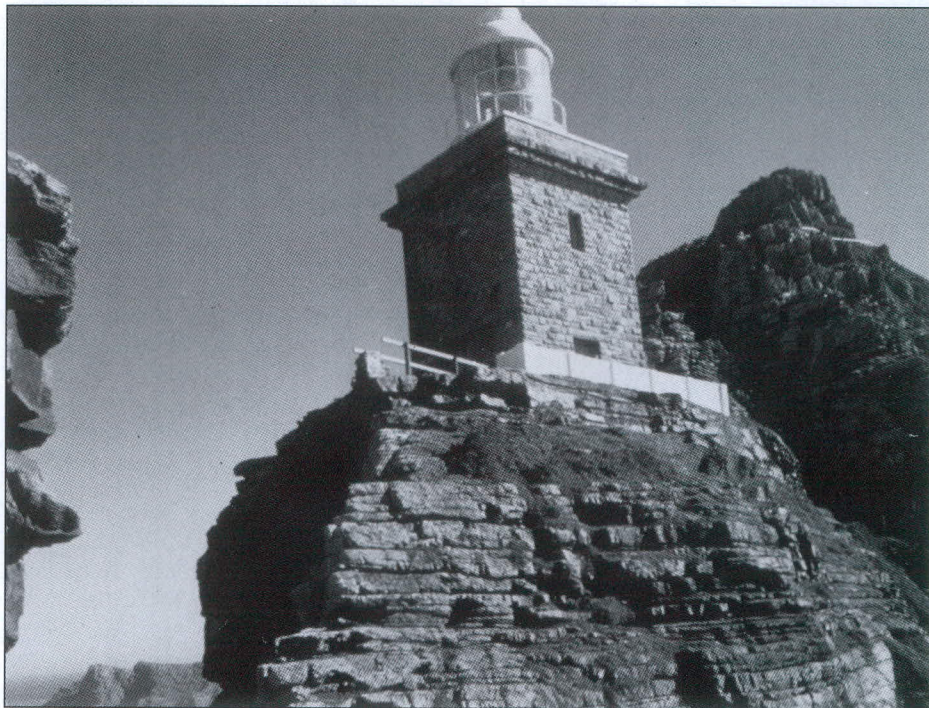
In 1914 the lighthouse at Cape Point was rebuilt 163 metres lower than the original. The large lens, heavy machinery and building materials were lowered with ropes and pulleys from the steep cliffs — an amazing feat of engineering for those days.
