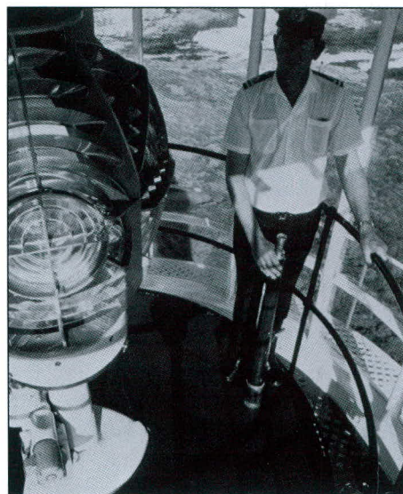
Senior keeper Koos de Kock on duty in the lantern room of the Danger Point lighthouse near Gans Bay. The Fresnel lens appears to be a 3 1/2 order. It is rated at one million candlepower.
