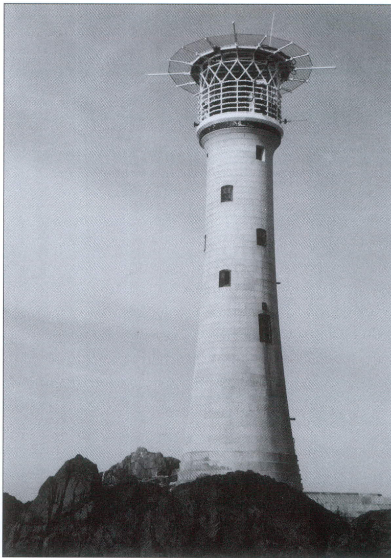
The Hanois Lighthouse in 1988. A helicopter landing platform has been placed on the lantern room. Photo by Keeper John Mobs.
