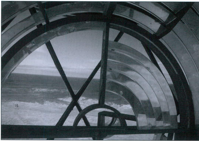
Above and below: Prisms are missing from the Fresnel lens, still in place in the tower.
