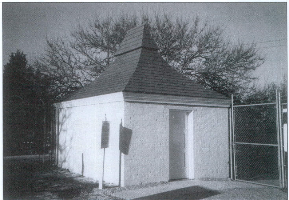
The brick oil house was constructed in 1893 after the station changed from lard oil to kerosene. The peaked roof is an unusual design for an oil house. The Mid Atlantic Center for the Arts restored this structure in 1990. It now houses the lighthouse orientation center and museum shop. Photo courtesy of MAC.
