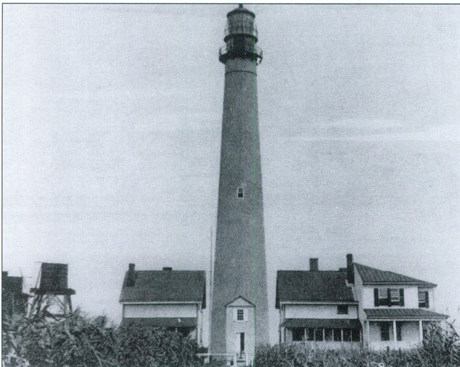
Above—Cape May Light Station shortly after the 3rd Assistant Keeper's quarters (far right structure) was built onto the side of the 1st Assistant Keeper's quarters. The 1902 addition ignores the architectural symmetry of the site. The wooden water tower, at left, stored water for the borough of Cape May Point. Photo taken from an old Post Card and courtesy of the Mid Atlantic Center for the Arts.
