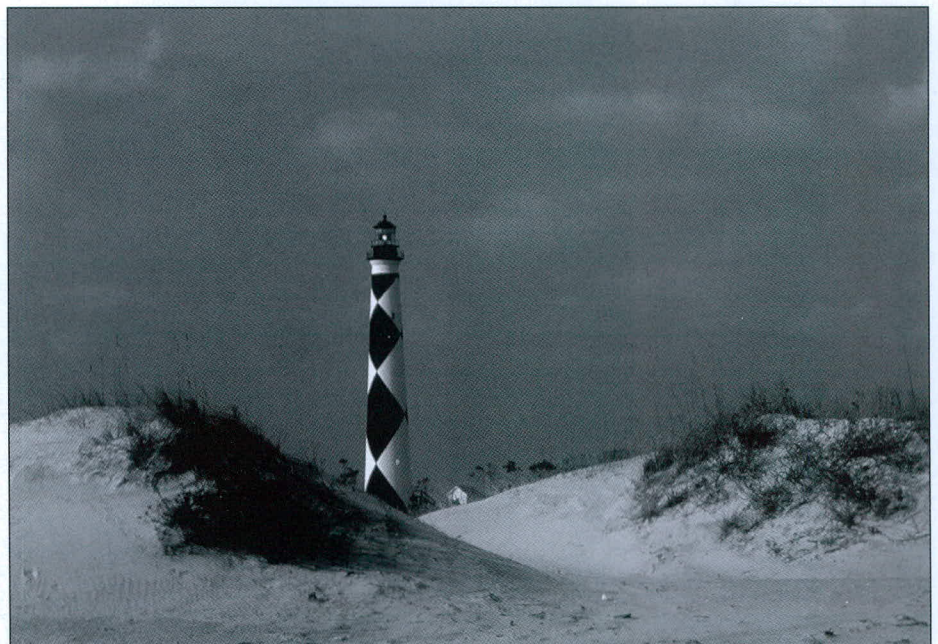
After 150 years of service, the lighthouse received repairs including replacing the exterior entry wood stairs and landing to match those constructed in 1859; strengthening the cast-iron spiral stair treads; repairing treads that were cut to install the 1916 clockwork mechanism to turn the first-order Fresnel lens; and replacing the handrail on the gallery, including adding safety mesh to make the gallery safe for children.
