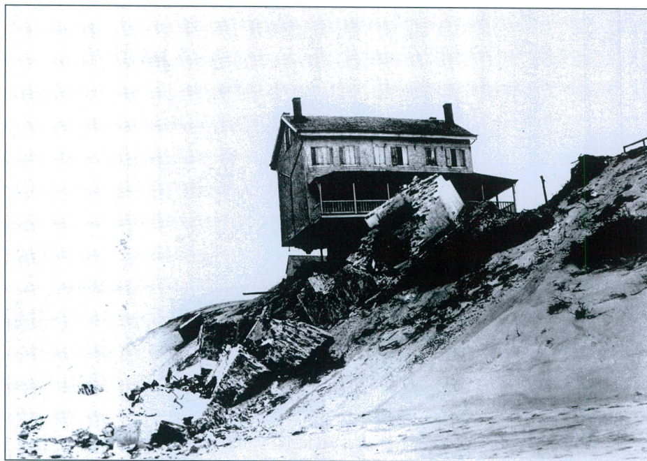
Aftermath of the storm of 1926. The ruins of the wrecked tower are in the foreground. National Archives photo.
