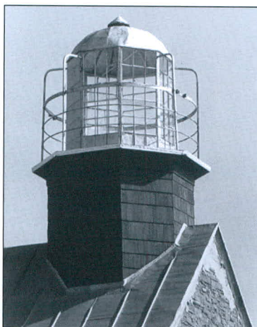
The lantern room of the Selkirk (New York) Lighthouse on Lake Ontario is one of the few old style "bird cage" lanterns remaining in the country. Photo from 1989 by Joel Lauterbach.
