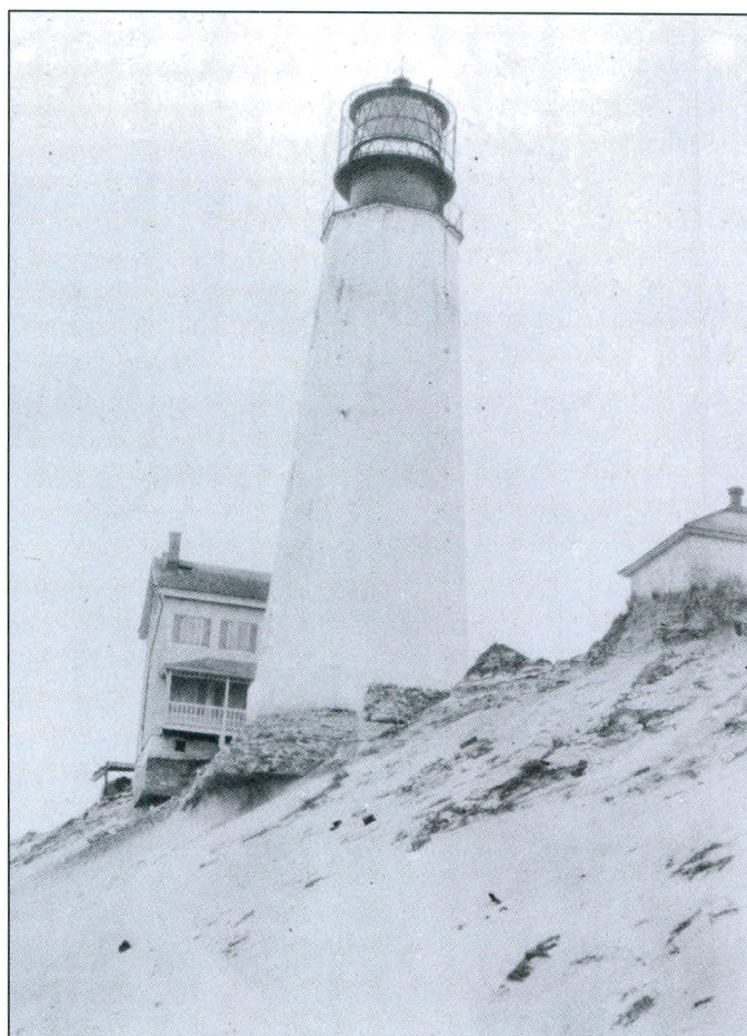
Below – left and right – Erosion undermines the keeper's house and the tower, circa 1925. Note that the lens has been removed from the lantern room in both photos. In the left photo the basement cistern has slid out from under the house and is halfway down the bank. U.S. Coast Guard photos.
