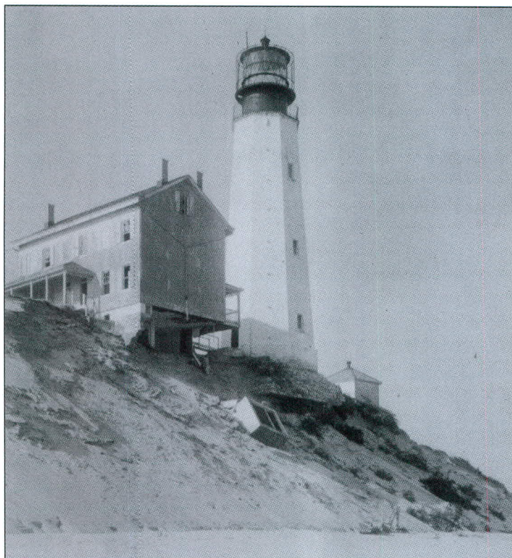
Below – left and right – Erosion undermines the keeper's house and the tower, circa 1925. Note that the lens has been removed from the lantern room in both photos. In the left photo the basement cistern has slid out from under the house and is halfway down the bank. U.S. Coast Guard photos.
