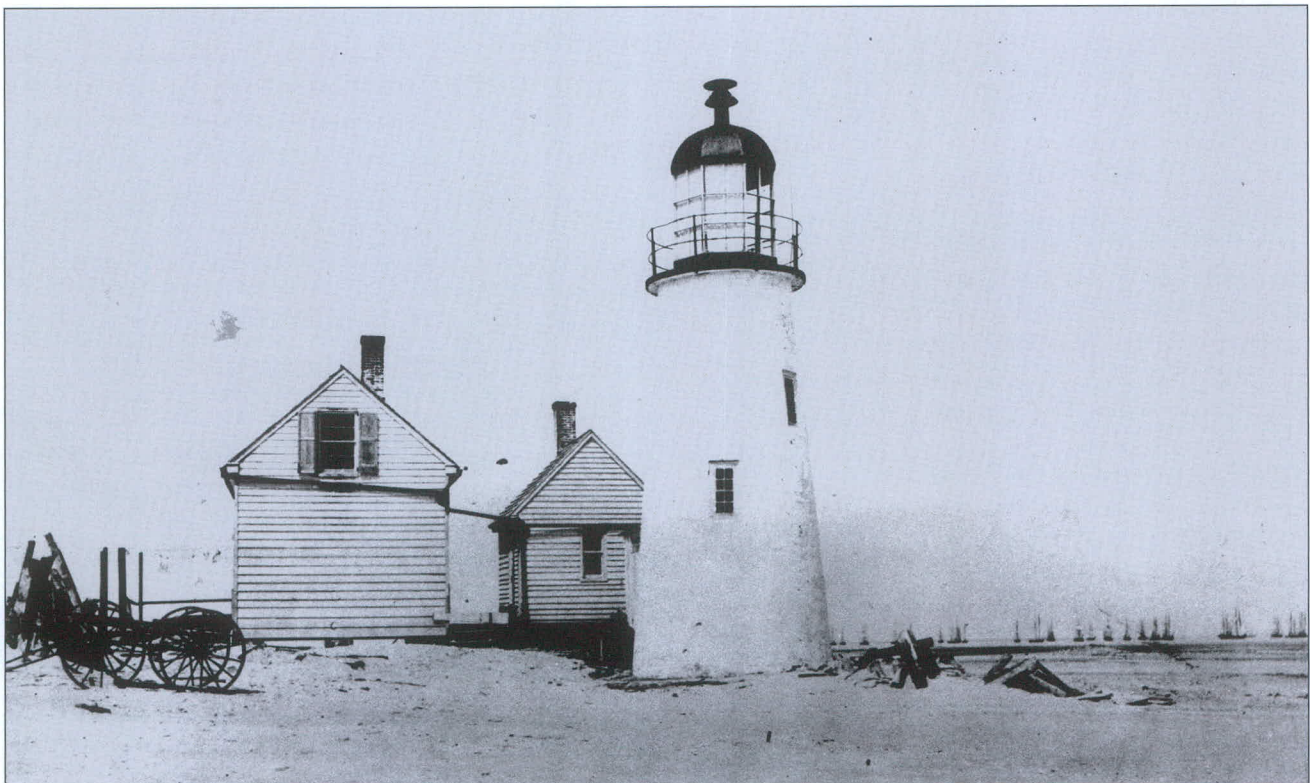
Cape Henlopen Beacon Light (constructed in 1825) in May 1863 shortly before it was torn down. Note the old-style lantern room with small panes and antiquated vent. A storage shed is next to the tower and the dwelling to the left. Note numerous ships in the background, possibly blockading the entrance to Delaware Bay. National Archives photo.
