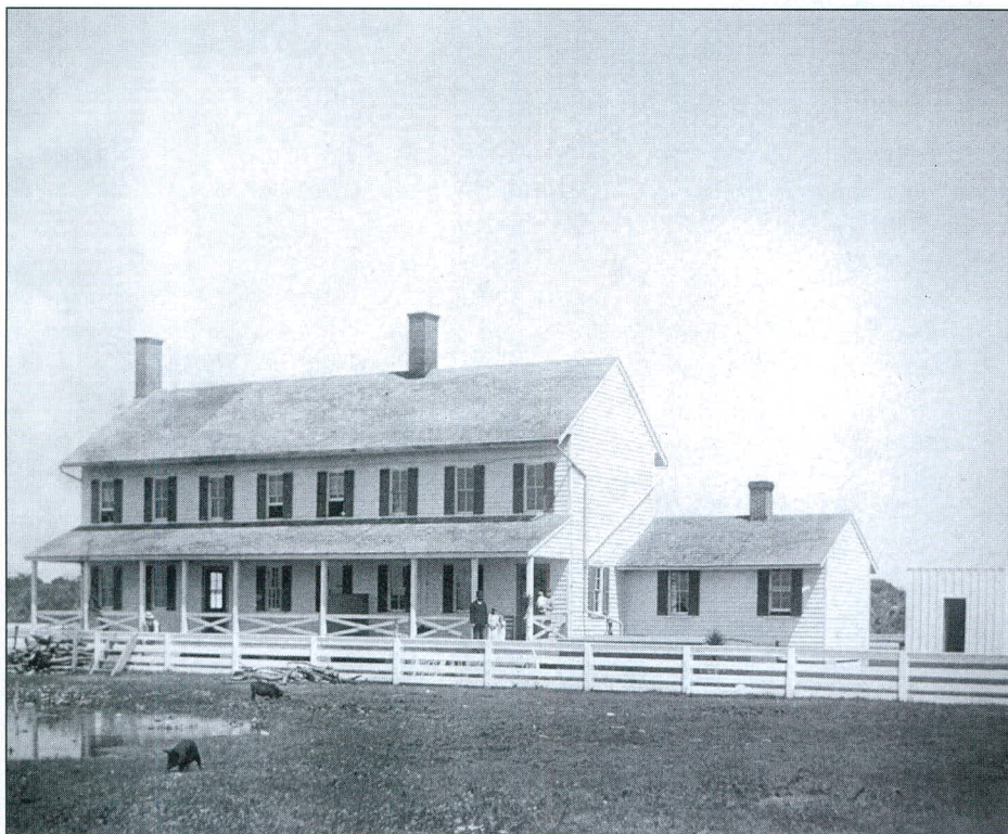
Above — The assistant keepers' dwelling circa 1894. Today this building is used for exhibits and as offices.
