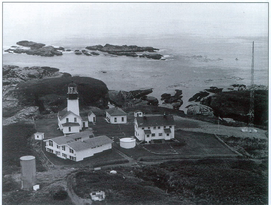
Cape Flattery Light Station showing the modern quarters left, old duplex center (right of the water tower) and the radio beacon antenna at far right. Photo courtest of the U. S. Coast Guard, August 8, 1974.
