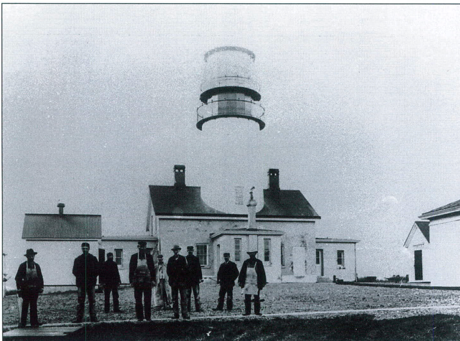
An 1872 photo of the workmen who constructed the fog signal building (at right) shortly after it was completed. Notice the granite of the lighthouse hasn't been painted yet. National Archives photo
