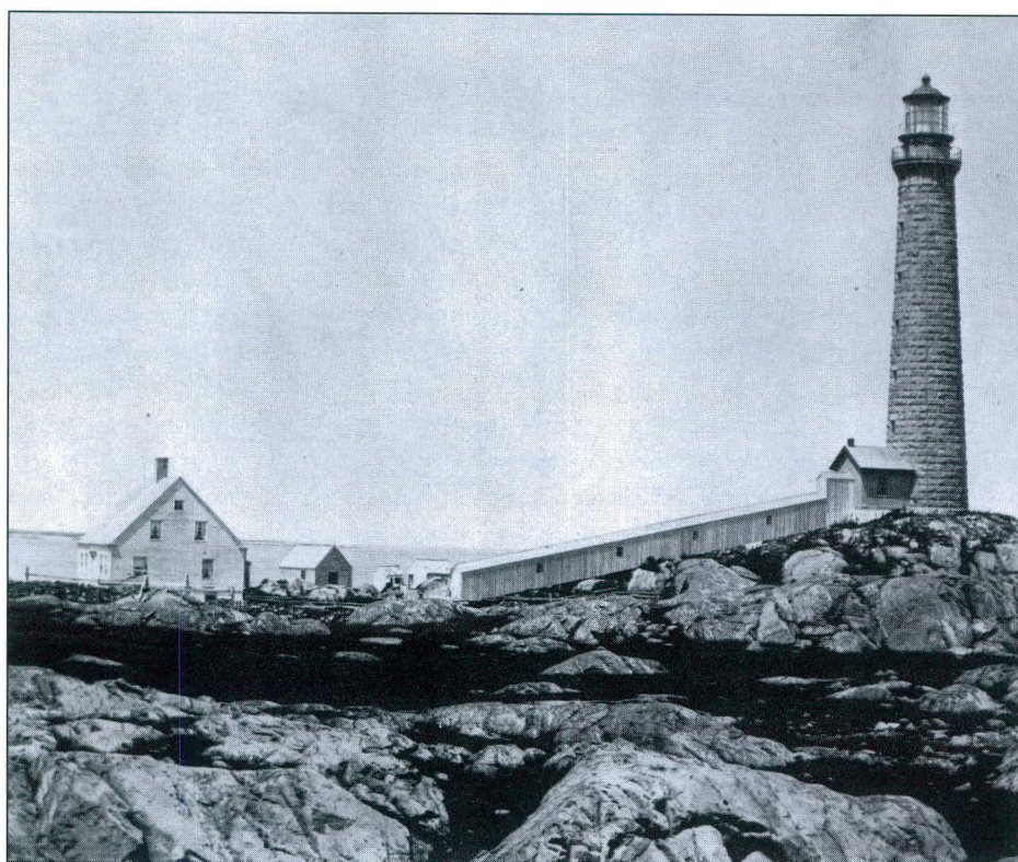
Above – Cape Ann Light Station's north tower with assistant keeper's dwelling at left. Note the long covered walkway to protect the keepers during inclement weather.
