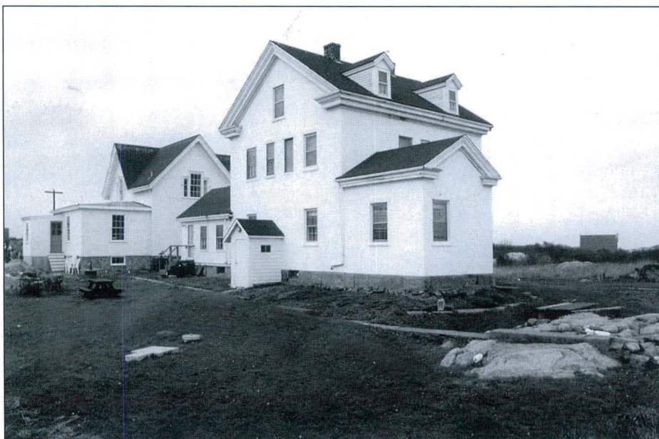
Cape Ann's duplex dwelling (foreground) and head keeper's dwelling. Photo courtesy of Thacher Island Association.
