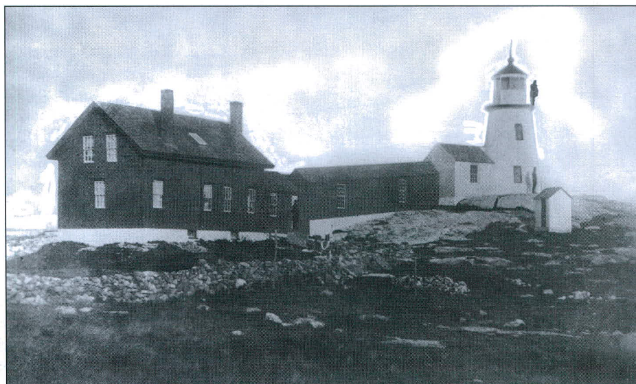
This view of the back side of Burnt Island Light Station circa 1858 shows dark vertical siding and a skylight in the roof. Note the three men; one at the back entrance of the dwelling, one at the foot of the tower, and another on the lantern deck. Photo courtesy of the U. S. Coast Guard.
