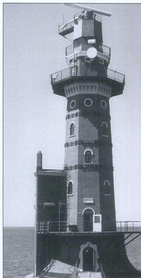
Above – Hoheweg lighthouse, constructed in 1856, is still in service today. The radar and microwave antennas on the top are the obviously recent adaptations. Photo courtesy German Maritime Museum, Bremerhaven.
