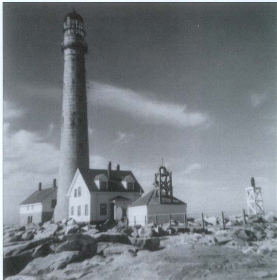
Boon Island, December 1961. Old, remodeled dwelling at left, newer dwelling in front of tower. Note bell on fog signal building and minor optic at far right. Photographer unknown.
