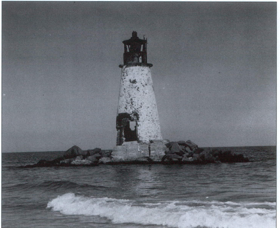
Below — The tower in 1950 all but destroyed by erosion. Note the rubble stone construction and old style lantern room. Photos courtesy of the author.
