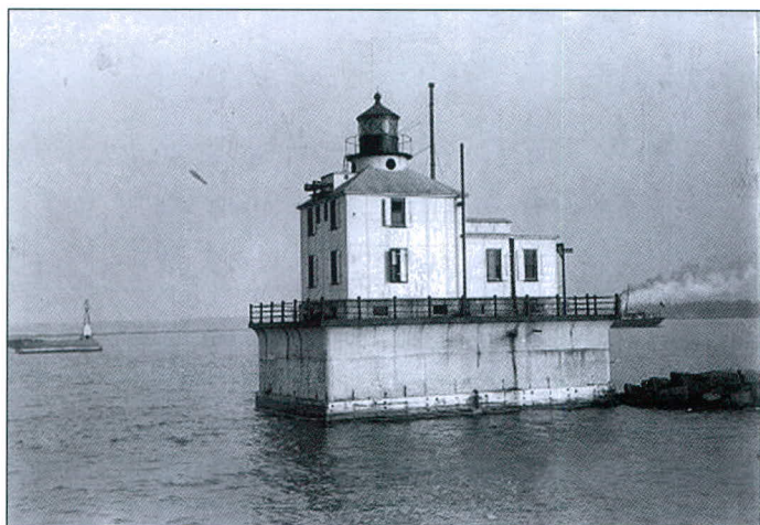
Ashtabula Light Station circa mid-20th century. Note the fog signal horns projecting from the dormer below the lantern. U.S. Coast Guard photo.
