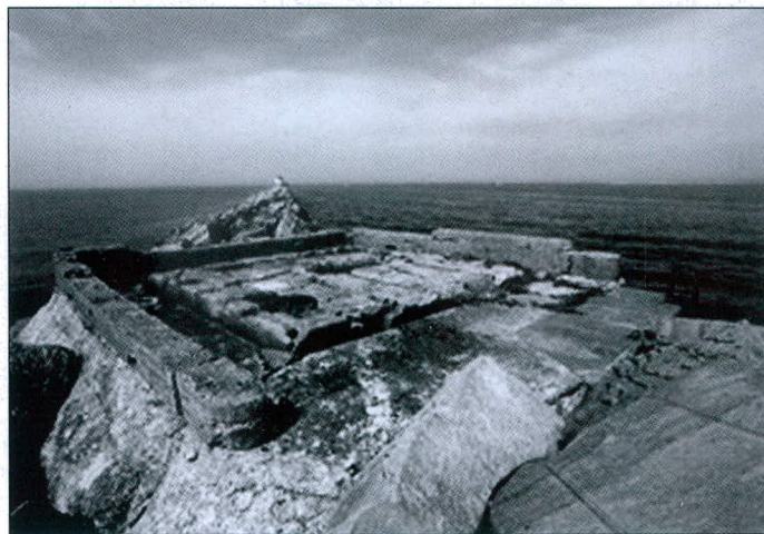
The remains of the original lighthouse foundation. Photo from author's collection.
