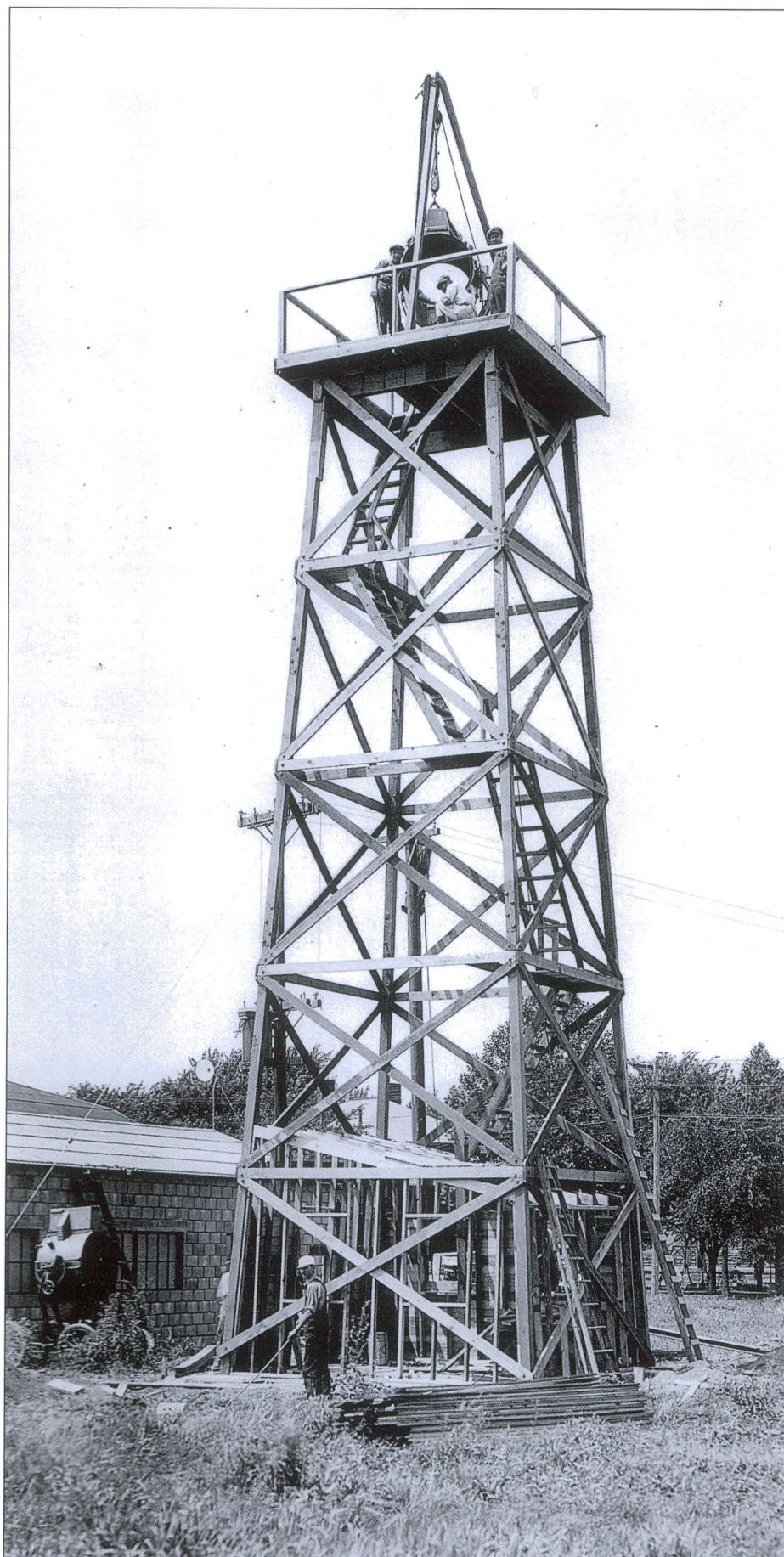
Installing an airways flood light.
