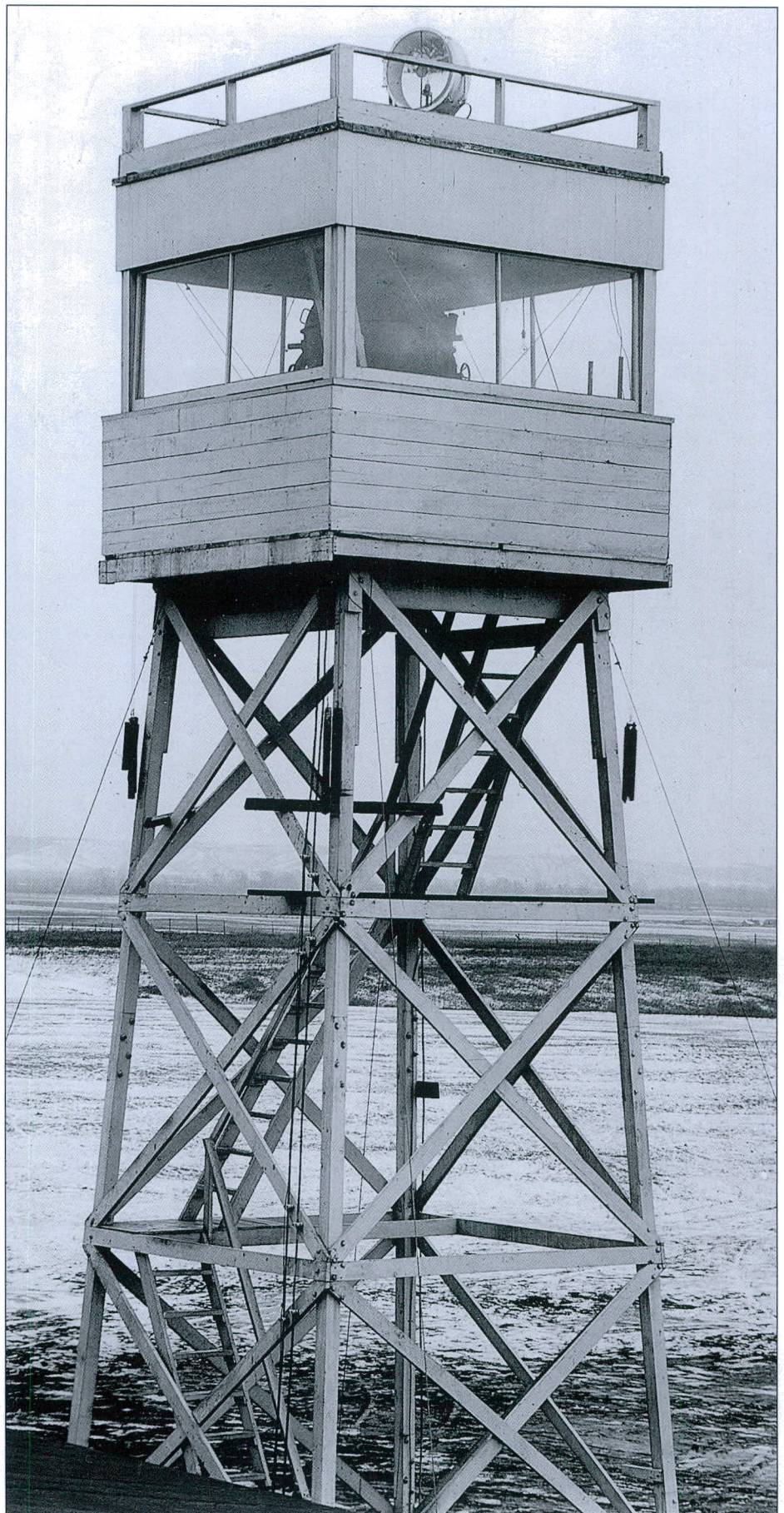
Tower holding flood light.
