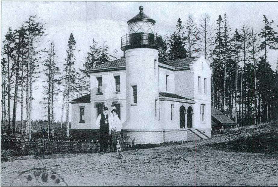
Above – The new Admiralty Head Lighthouse shortly after construction from an old Post Card dated 1907. Right – The restored Admiralty Head Lighthouse in 1984. Note that the replacement lantern has vertical astragals (bars between the glass storm panes) in lieu of the diagonal astragals of the original lantern. The gallery railing and ball vent closely resemble the originals. Photo by Fred Stanio.
