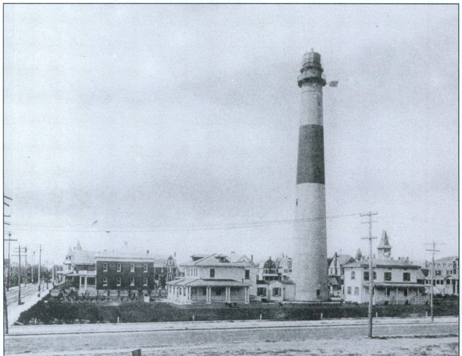
The Absecon Light Station in 1909. The station encompasses an entire city block. The head keeper's house is at left, with a connecting passage to the tower. Until about 1908 the keeper's house had three stories (see photo on page 7). The assistant quarters is at right. National Archives photo courtesy of Keeper Robert Lewis.
